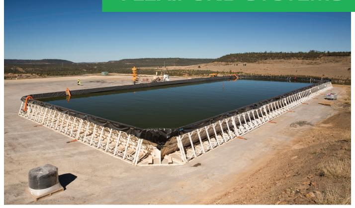
MPC Kinetic has developed patented FlexiPond technology to assist with above ground oil field fluid management, significantly reducing excavation costs.
